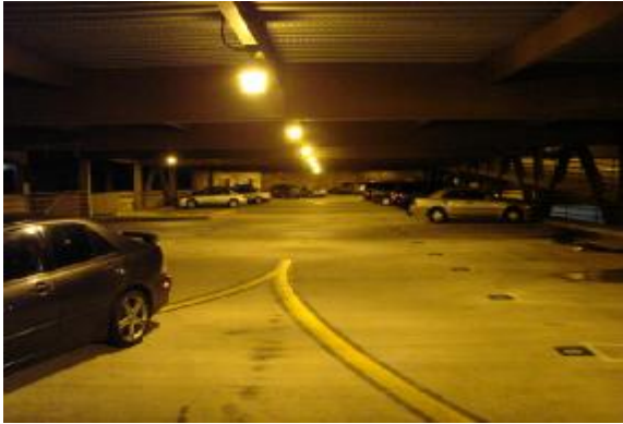
Before: 175W High Pressure Sodium
