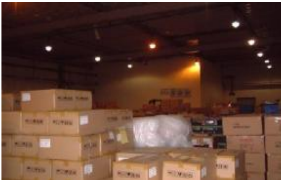
Before: 175W HPS and 150W Metal Halide
